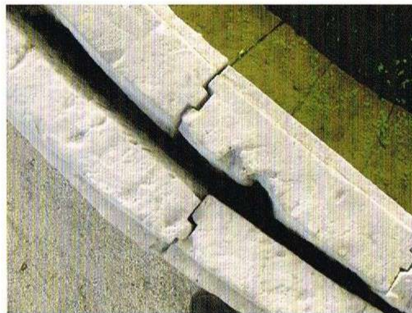
Image 7: Examples of coral stone interlocking joinery from early modern period
